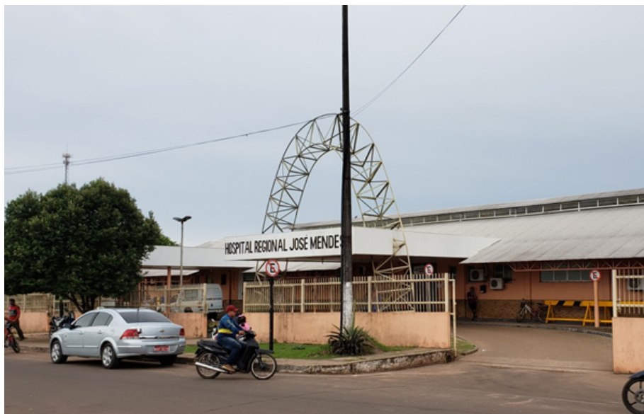
Figura 2 - Fachada do Hospital Regional José Mendes, Itacoatiara, Amazonas, Brasil
