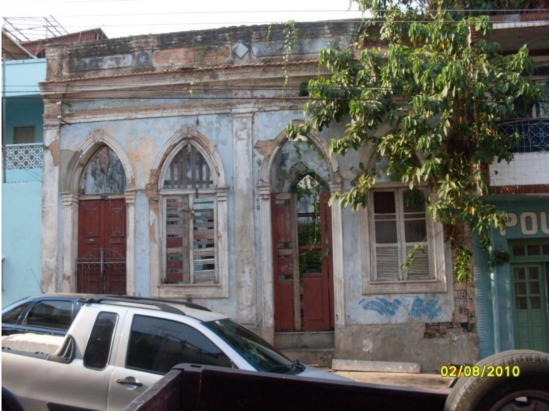
Rua Miranda Leao, 475
